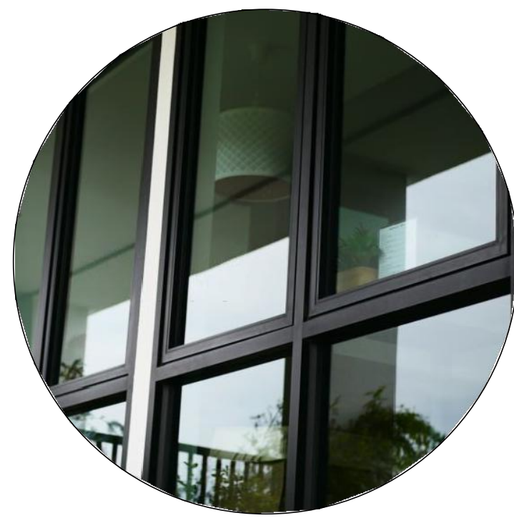
4 TINTED GLASS FOR STOREFRONTS, WINDOWS, BALCONY DOORS VIRACON - 9/16" VLE24 - 47 LAMINATED HS/HS
